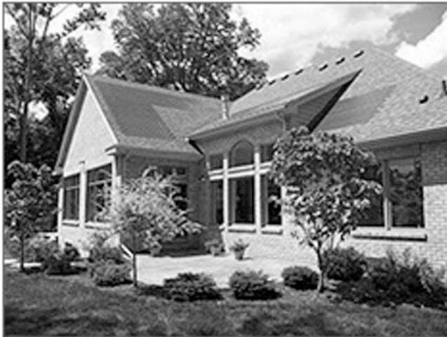
Figure 4.3 A home's roof using thin-film solar tiles.
